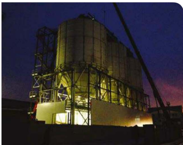
Due to the latitude, the daylight was very short requiring a proper illumination plant.
