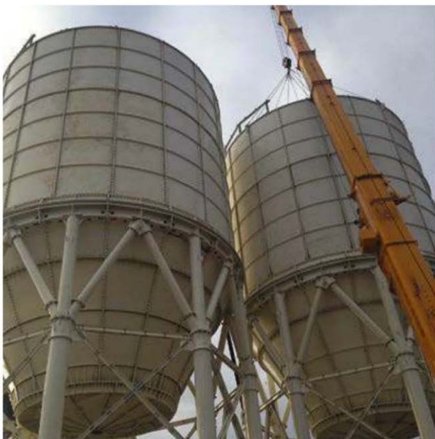
Two of the three silos almost erected, showing the discharge cone installed on the carrying structure.
