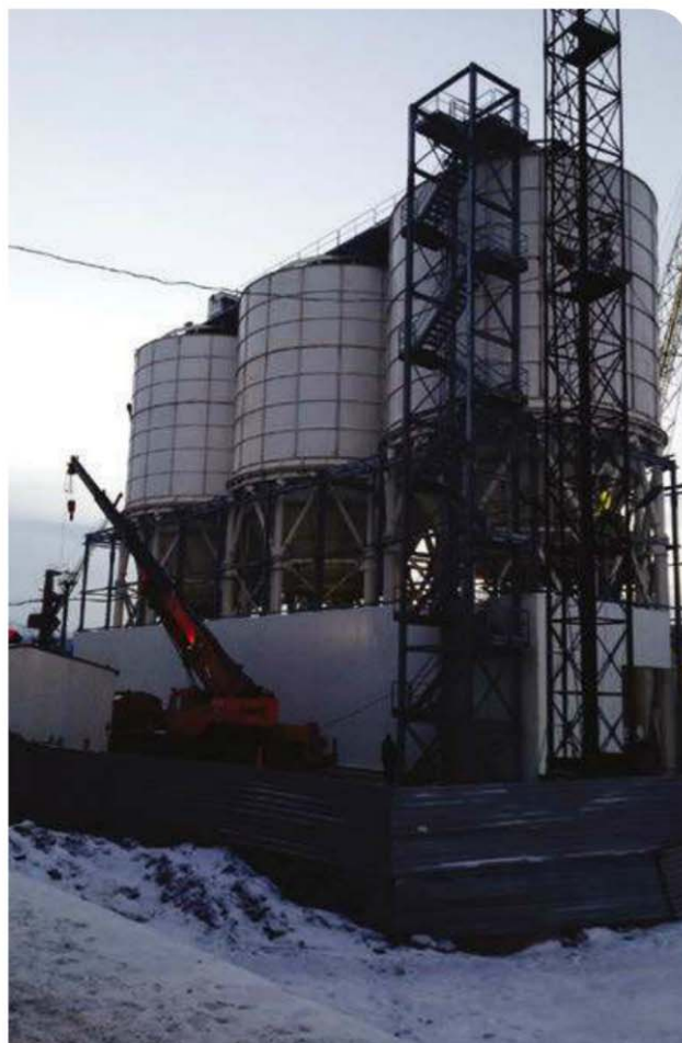
Installation progress in September, when it started snowing.
