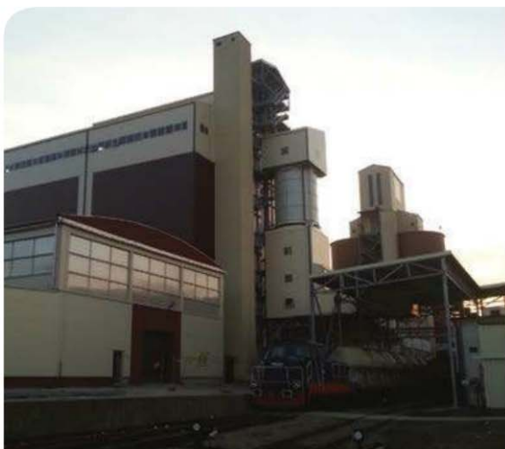
Figure 2. General view of the project facility, which is in line with the architectural style of the neighbourhood.
