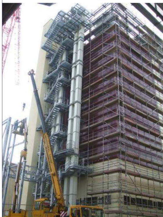
Figure 5. Above: installation of the components at the narrow site; below: a 3000 \text{ m}^2 scaffolding was erected while installing the housing.
