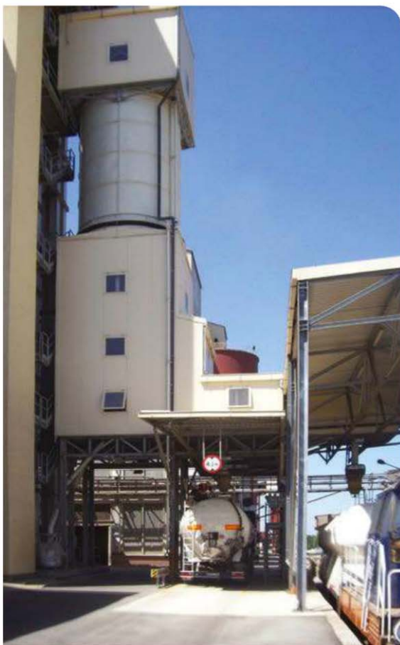
Figure 4. The cement loading stations.
